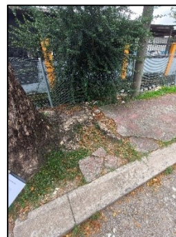
Figure 6. Cracks and uneven surfaces pedestrian path
