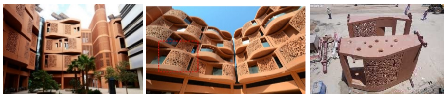
Figure 11 (a). The Residential Units in Masdar City having Mashrabiya on the wall and balcony.
