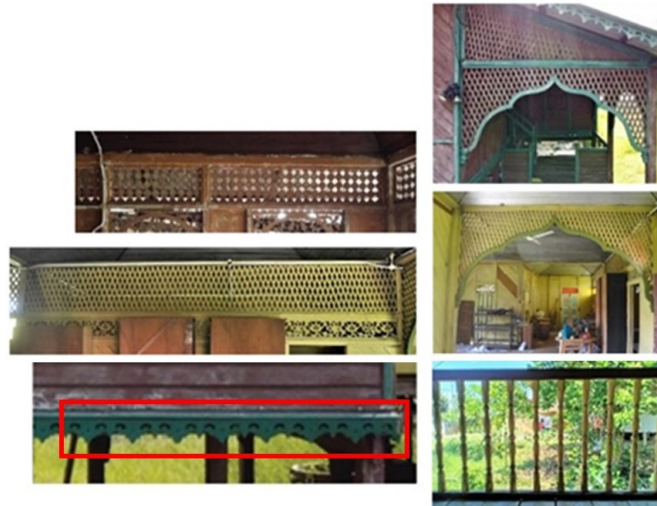
Figure 4: Gerbang Luar, Gerbang Dalam, Pagar Musang Serambi, Papan Manis, Lubang Angin Luar, and Lubang Angin Dalam (clockwise)
