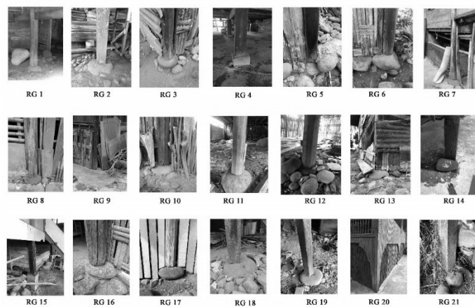
Figure 9: Elements of the Foundation Source: Desy Aryanti, 2021
