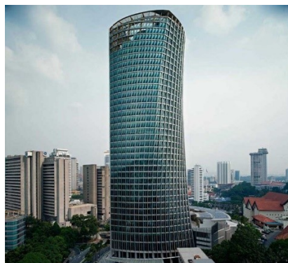
Figure 6: Public Work Department Block G (PWD) Source: 2017, KCJ Engineering SDN. BHD.
