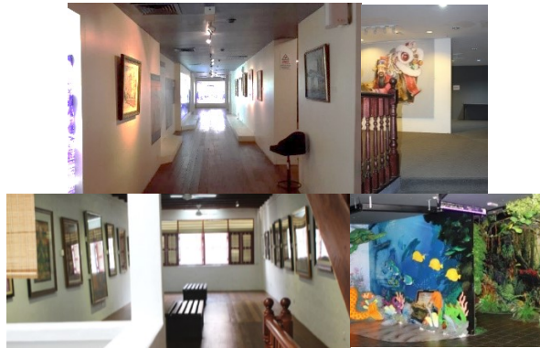
Figure 3: Insensitive installation of partitions, removal of original wall and extensive wall decorations were among the inappropriate physical interventions found involving internal wall element.
