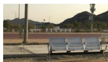
Figure 4.6: Aluminum bench material is unsuitable for hot and humid climate
