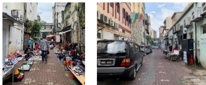
Figure 4: Condition of Lorong Petaling.
