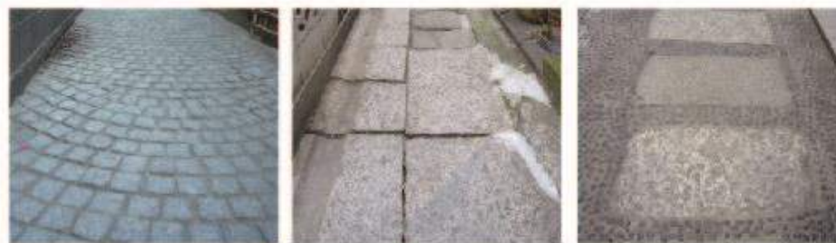
Figure 8: Types of Stone Pavements seen in Kagurazaka (Left is the Pinkoro pavement)
