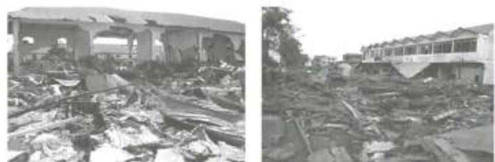
Figure 3: Tsunami effects in Banda Aceh earthquake, 2004
