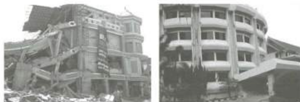
Figure 2: Ground shaking effects in Banda Aceh earthquake, 2004
