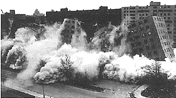
Figure 2: The Pruitt-Igoe housing development had to be torn down, at a loss of US$300 million, after it was declared unfit to be lived in. (Source: Newman, 1996, pg. 12)
