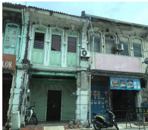
Figure 1: Heritage building that had undergone renovation
