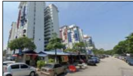
Photo 4: PPR Pantai Ria residential building
