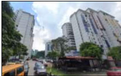
Photo 3: PPR Kerinchi Lembah Pantai residential building
