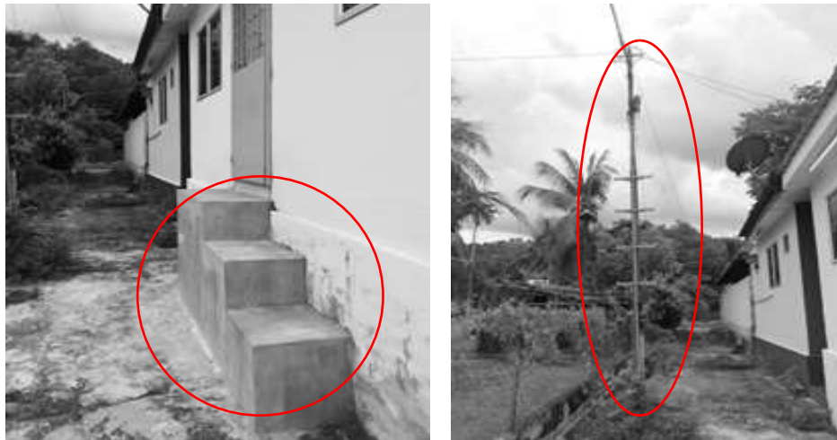
Figure 6: Stairs and utility poles become a tool for criminals to break into houses
