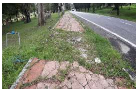
Photo 2: The poor condition of jogging track
