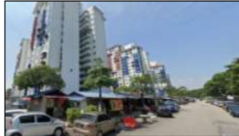
Photo 4: PPR Pantai Ria residential building
