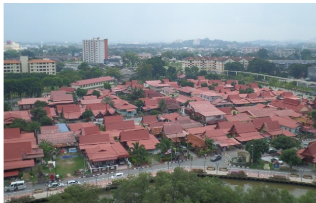
Figure 3: Most houses in Kampung Morten have undergone major renovations for the main structure, walls, windows, roofs and stairs since the year 2000
