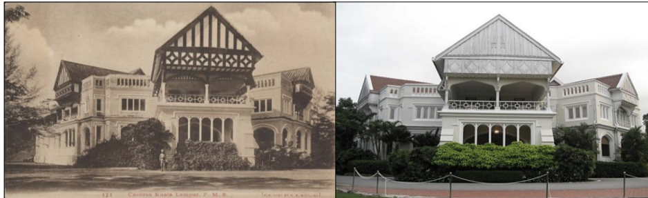
Figure 1: Carcosa in year 1900 (left) and the building in 2018 (right), still remain the original form and design, however the decorative timber at front gable has been painted and covered the Tudor features.
