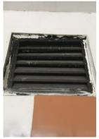
Figure 3 Unclean ducting system and stained floor, ablution room Gate-B
