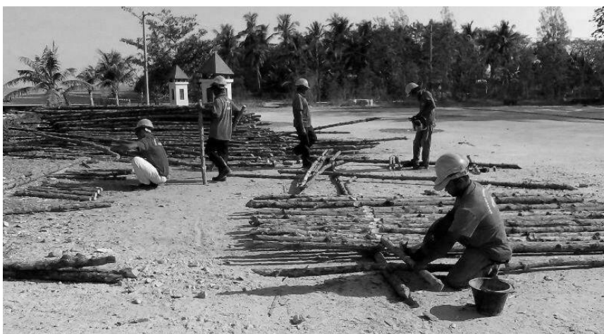
Figure 3: View of on-site construction works Source: Author
