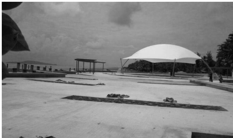
Figure 2: View of NCIA-AMB Project after completion Source: Author
