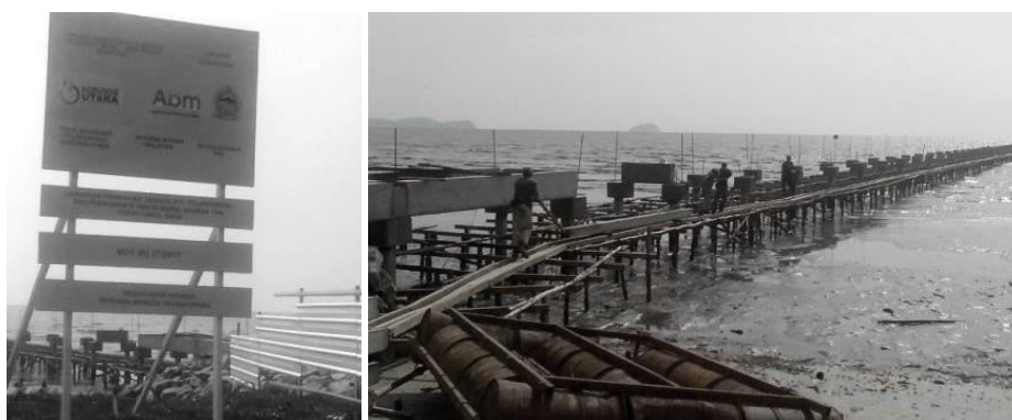
Figure 1: Execution stage of NCIA-AMB Kampong Project Source: Author
