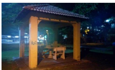
Photo 3: Lack of lighting at gazebo
