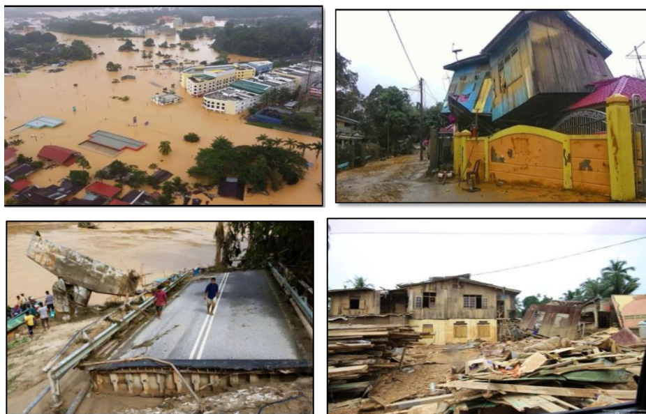
Figure 1: Views of study area when it was flooded in December 2014
