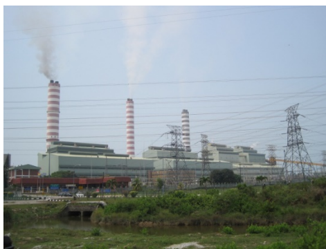
Figure 2: Example in Klang District: A factory plant located within coastal area creates conflict use.
