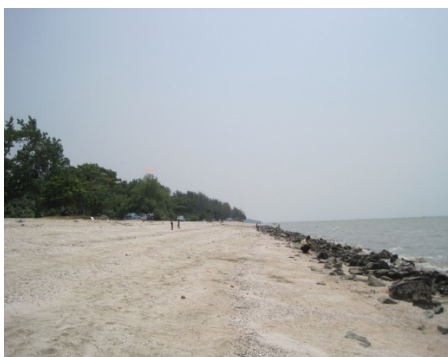
Figure 1: Pantai Remis in Kuala Selangor district is facing erosion problem that requires coastal defence work to curb it.
