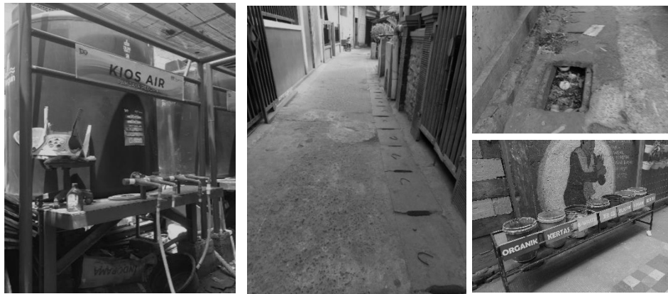
Figure 4: The Condition of Settlement Infrastructure Source: Author's Documentation
