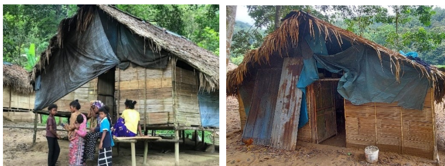
a) Canvas we used on the wall; Raised floor using bamboo
