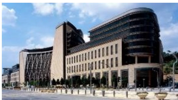
Figure 7: Exterior of the Ministry of Finance Source: (GDP web, 2020)
