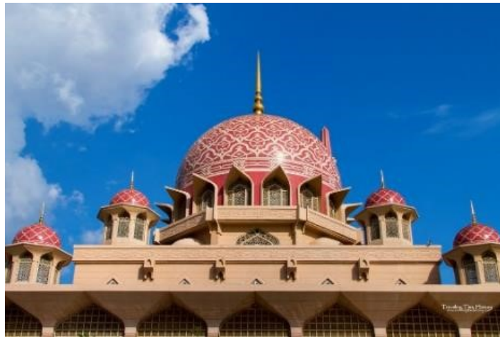
Figure 5: exterior view of Putra Mosque Source : (Adams, 2013)
