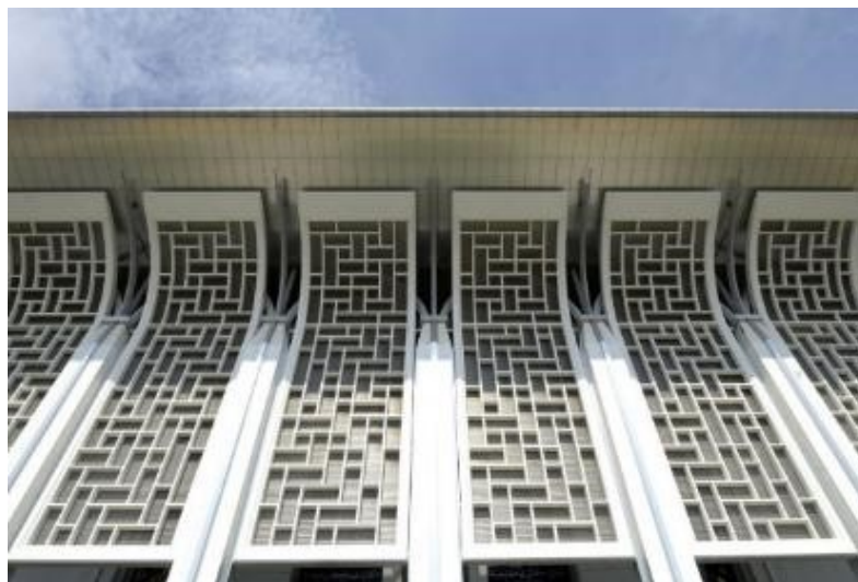
Figure 12: the stainless-steel spiral mesh at the back of the rectangular pattern Source : (GKD, 2019)
