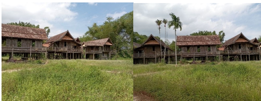
Figure 1: Condition of Pura Tanjung Sabtu that has been abandoned.
