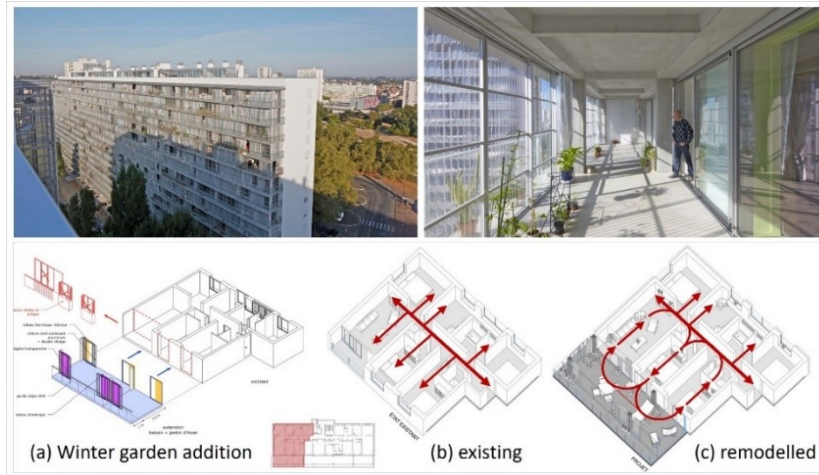
Figure 2: Fine-grained circulation and activity distribution by addition of winter gardens in the front facade of Bordeaux social housing in France
