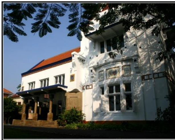
Figure 1 The Façade of CCCL Surabaya
